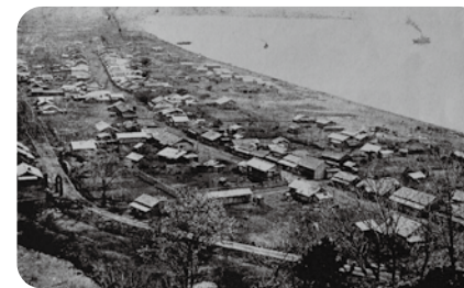
The Honcho district in 1906; in the top right of the photo, a smoking steamboat can be seen. Around the turn of the 19th century, Abuta rapidly developed as a stopover for pioneers arriving from mainland Japan.
