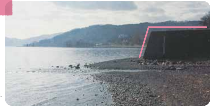
The volcanic ash was transported to the lakeshore, where an embankment was created.
